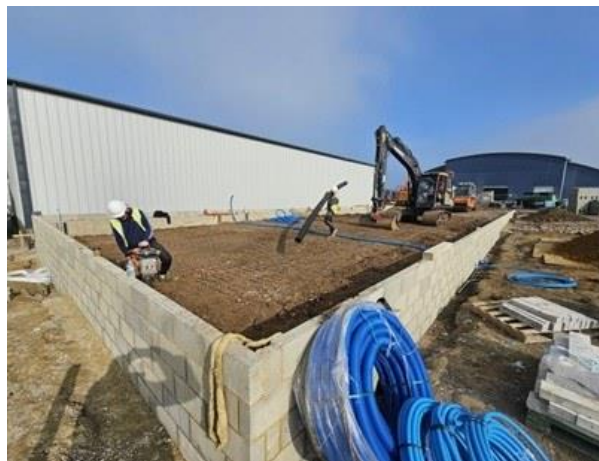
4 - Works underway at Manston Business Park
